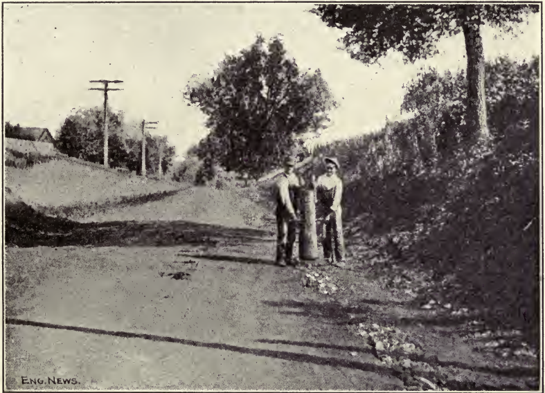
FIG. 6.—MACADAM ROAD ON STEEP GRADE, WITH SHALLOW-PAVED GUTTERS.
